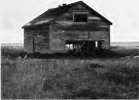
FIGURE 1. Abandoned building containing Black Guillemot nests, Herschel Island.
