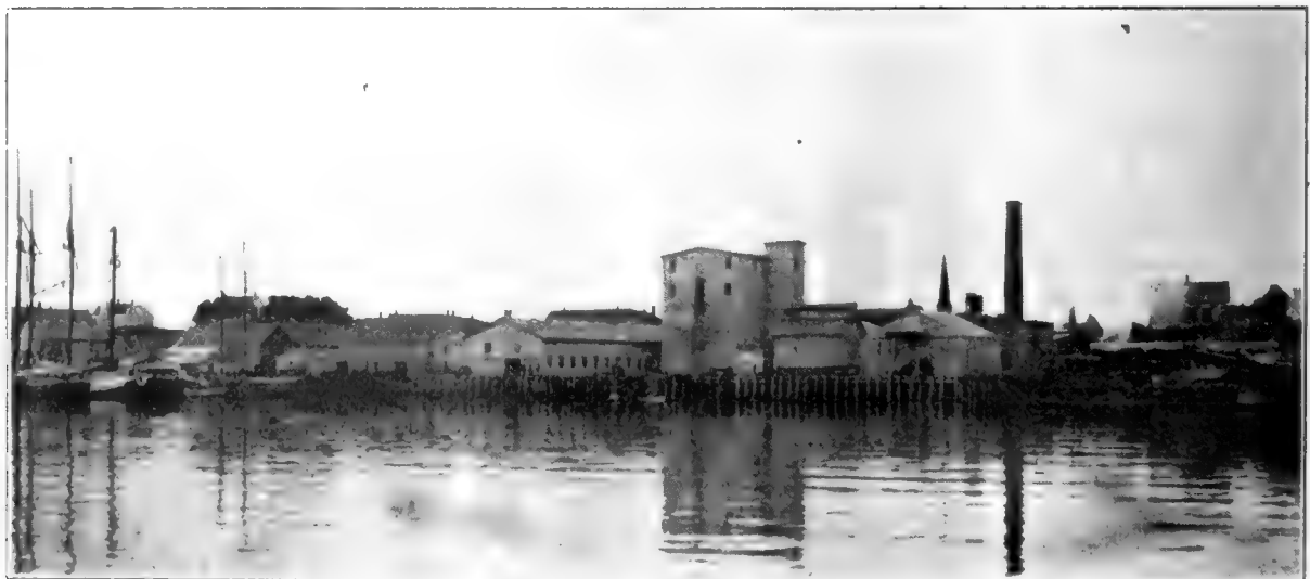
The Plant of the Lockeport Cold Storage Co., Ltd., Lockeport, Nova Scotia.
