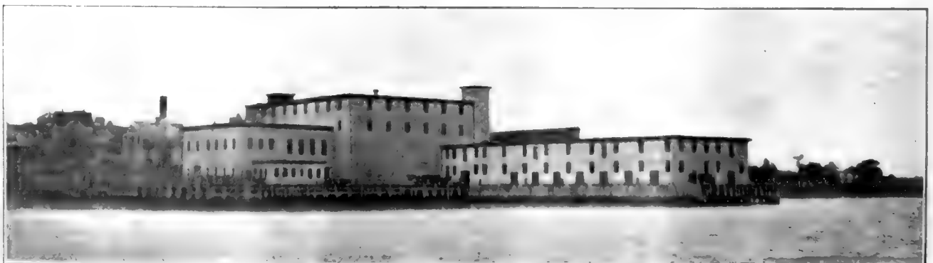
View of Plant from Water.
