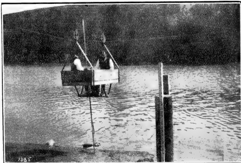
Photo by P. M. Sauder, 190 Cable Car and Gauge Height, Elbow River, Alta.
