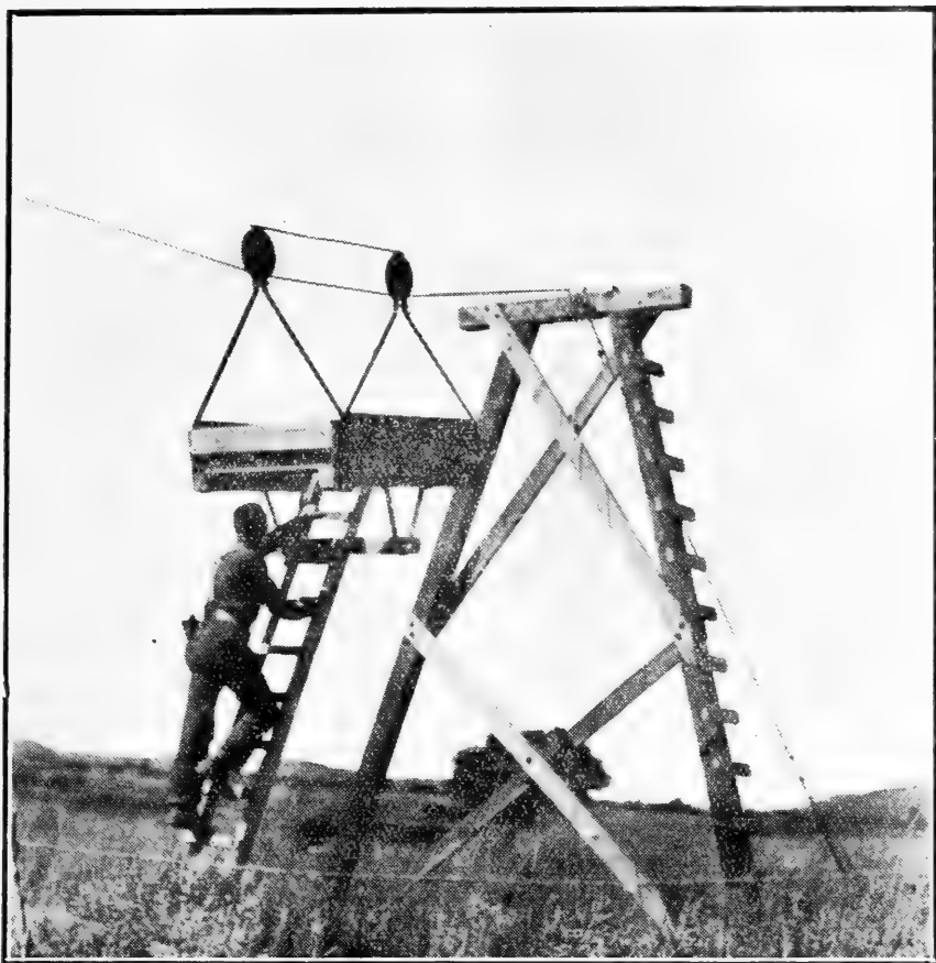
Cable Car and Frame Complete.
