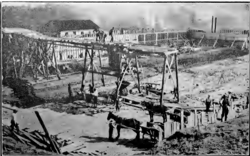
Erecting Abitibi Pulp Co. plant, Northern Ontario.
