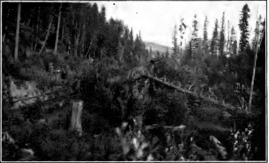
Railway right of way previous to clearing. The Railway Act requires that railway rights of way shall be maintained free from combustible matter.
