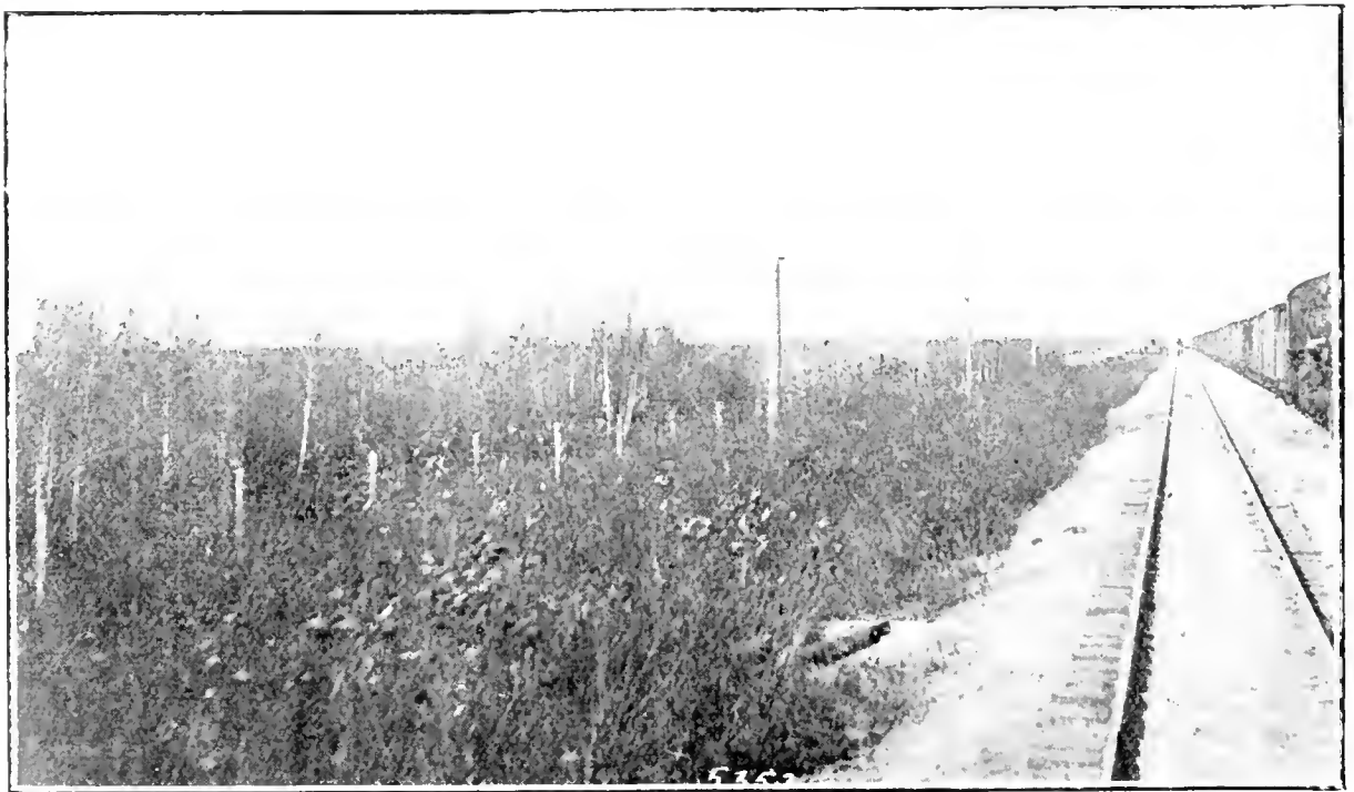
Another kind of right-of-way. Here the ground has received very little attention. The grass and shrubbery are in an ideal condition for fire.
