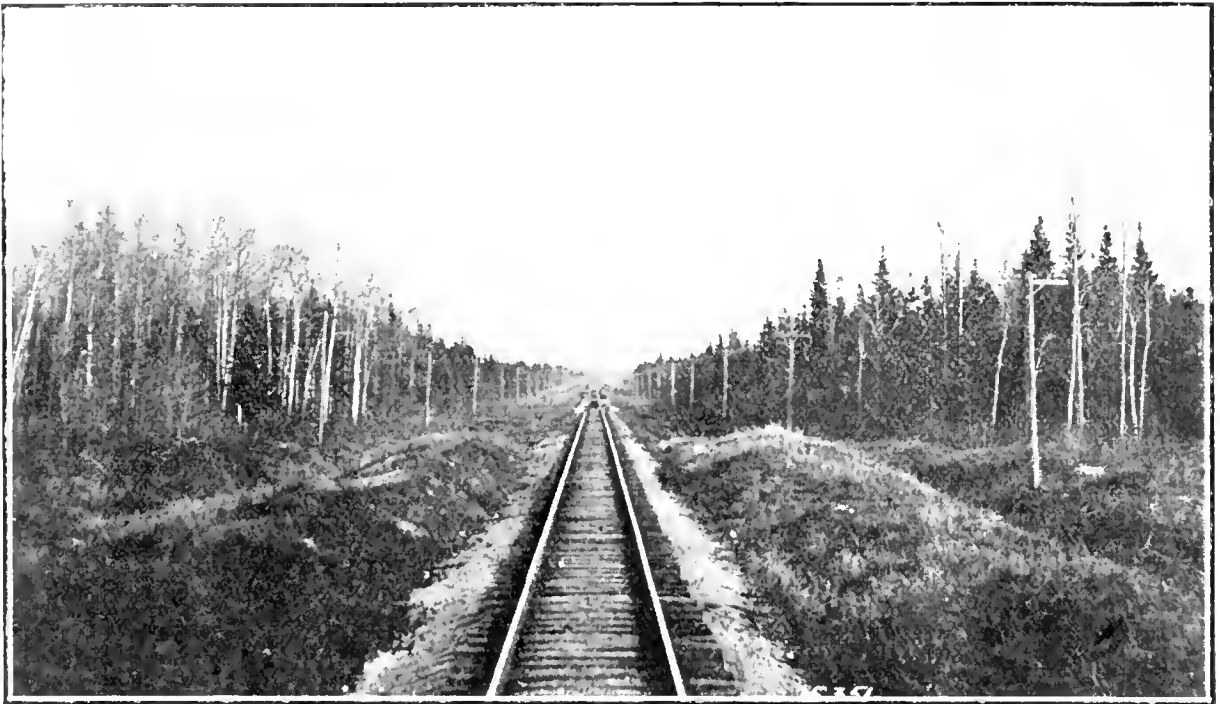
A Canadian railway right-of-way well cleared and presenting a minimum fire risk.
