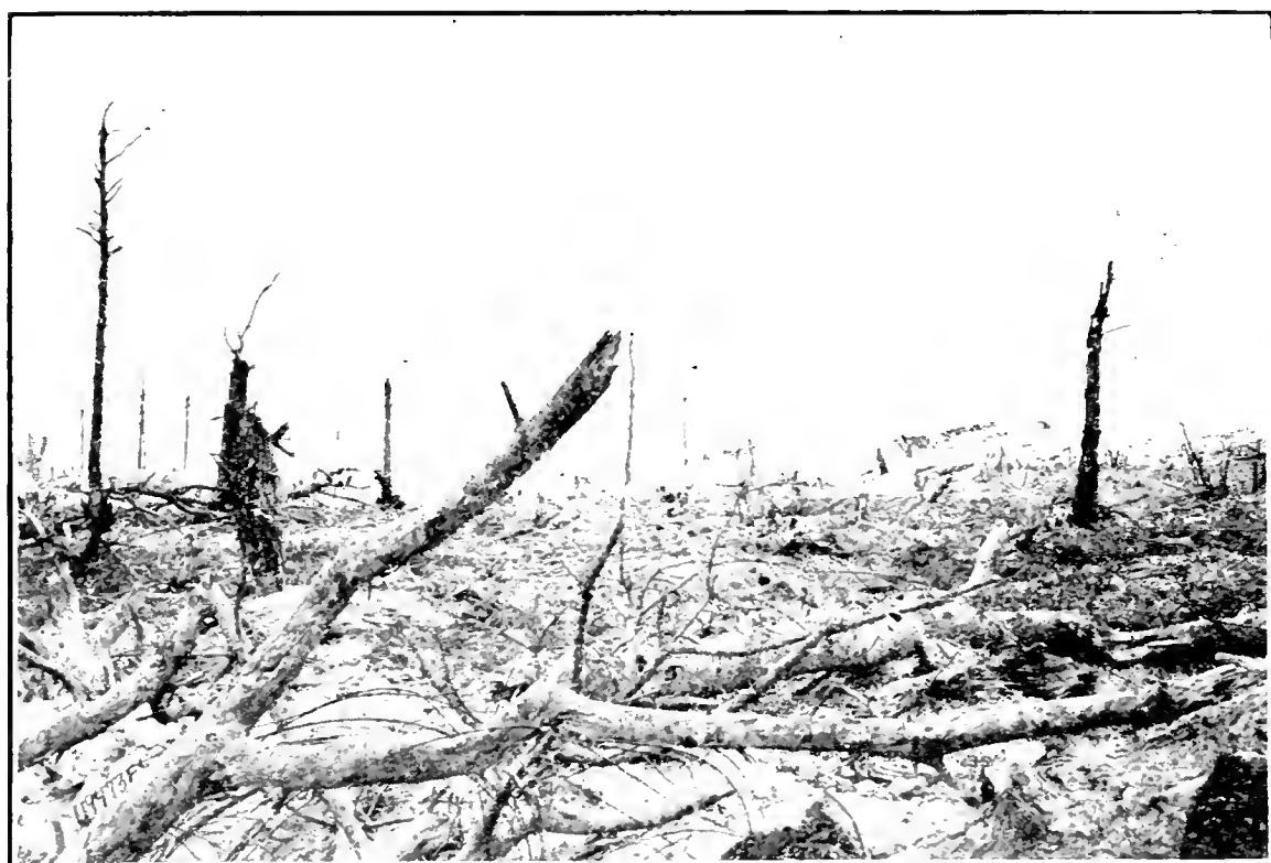
French first line trenches plowed by German shells. The forest in this section was battered to fragments.
