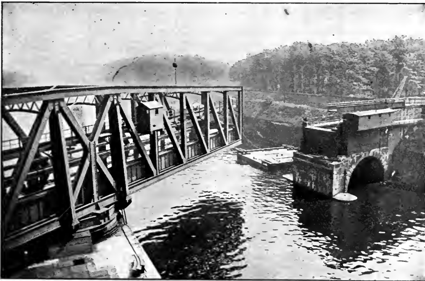
AQUEDUCT BEING SWUNG ASIDE TO ALLOW VESSEL TO PASS ON SHIP CANAL BENEATH
