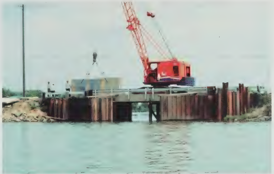
Figure 18.12. The control structure between North and South Spring Lakes under construction.
