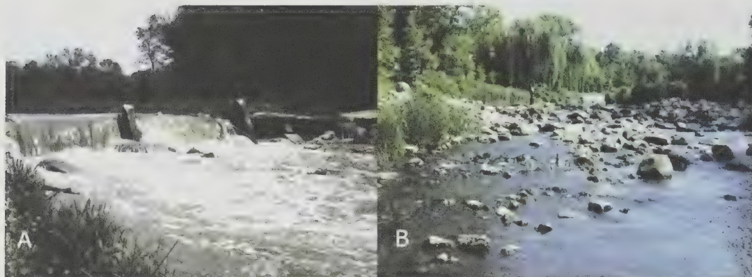
Figure 18.4. Removal of a dam on Waubensee Creek in Kendall County. Replacement of the dam with a constructed riffle allows fish passage. A) before, B) after. Photos by J. Rodsater.
