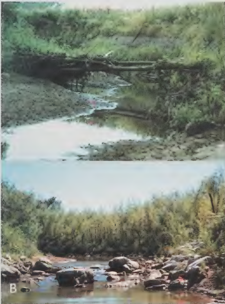
Figure 18.2. Example of a bank stabilization and instream habitat improvement project on Cox Creek in Cass County. A) Site before start of project. Note the steep bank and lack of a buffer between the bank and rows of corn. This site has low aquatic habitat diversity. B) Post-construction. The willows on the bank absorb energy generated by water during high flows, thus reducing bank erosion. The lunker structures at the base of the streambank provide a habitat for larger fishes. In the foreground, constructed rock riffles create habitat for riffle-loving fishes and invertebrates.
