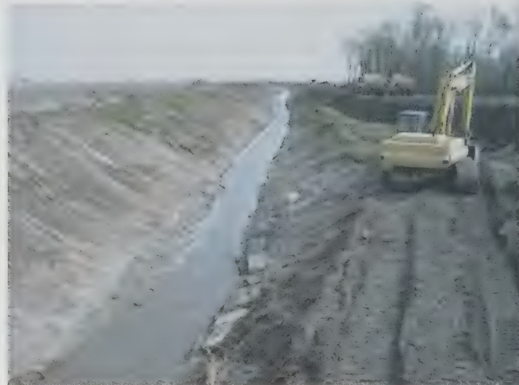
Figure 5.2. Typical trapezoid-shaped dredge channel just after completion. Note the clearance of riparian vegetation. Photo by C. Bullard.
