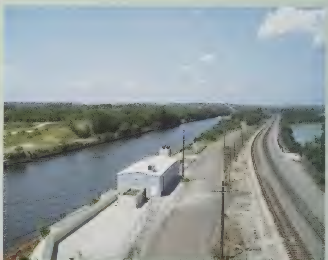
Sidebar Figure 3. This non-descript building found along the Chicago Sanitary and Ship Canal in northeastern Illinois houses the equipment necessary to maintain an electric dispersal barrier. Photo by P. Moy.
