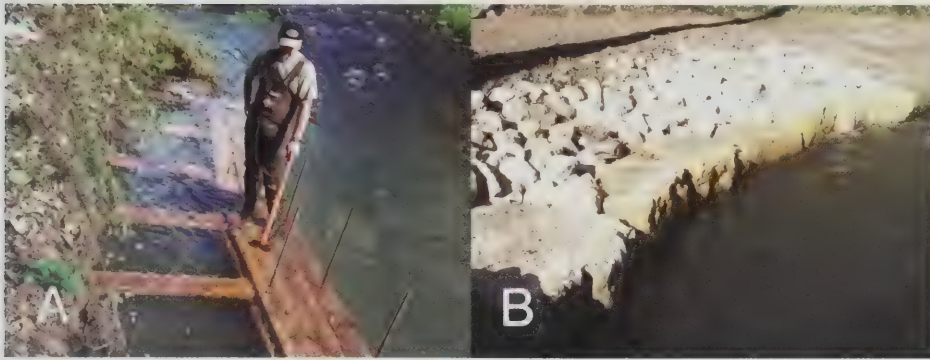
Figure 18.1. Example of a bank stabilization and in-stream habitat project in northwest Illinois. The wood structure A) is a lunker structure, which creates an overhanging bank for fishes. B) The lunker structure and streambank are stabilized by the addition of rock. Photos by K. Rivera.
