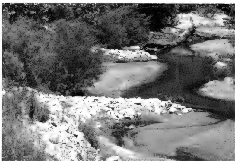
Figure 18.5. An example of bendway weirs. Note that the weir moves the thalweg (the deepest part of the channel) away from the eroding bank.
