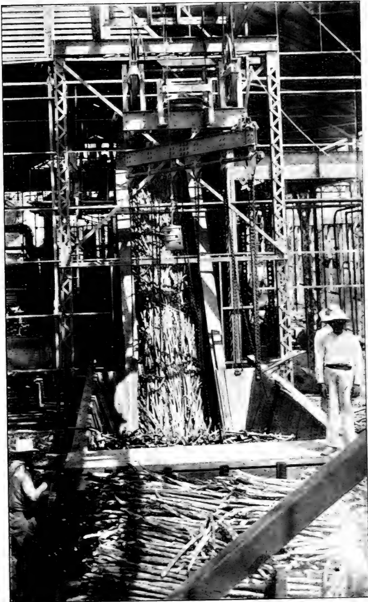
CANE HOPPER AND ELEVATOR.
