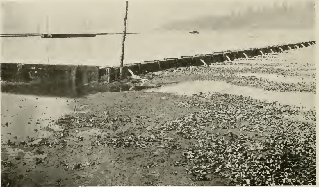
METHOD OF DIKING OYSTER GROUND EMPLOYED ON PUGET SOUND, WASH.
