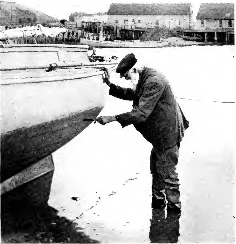
Hunting for a leak
