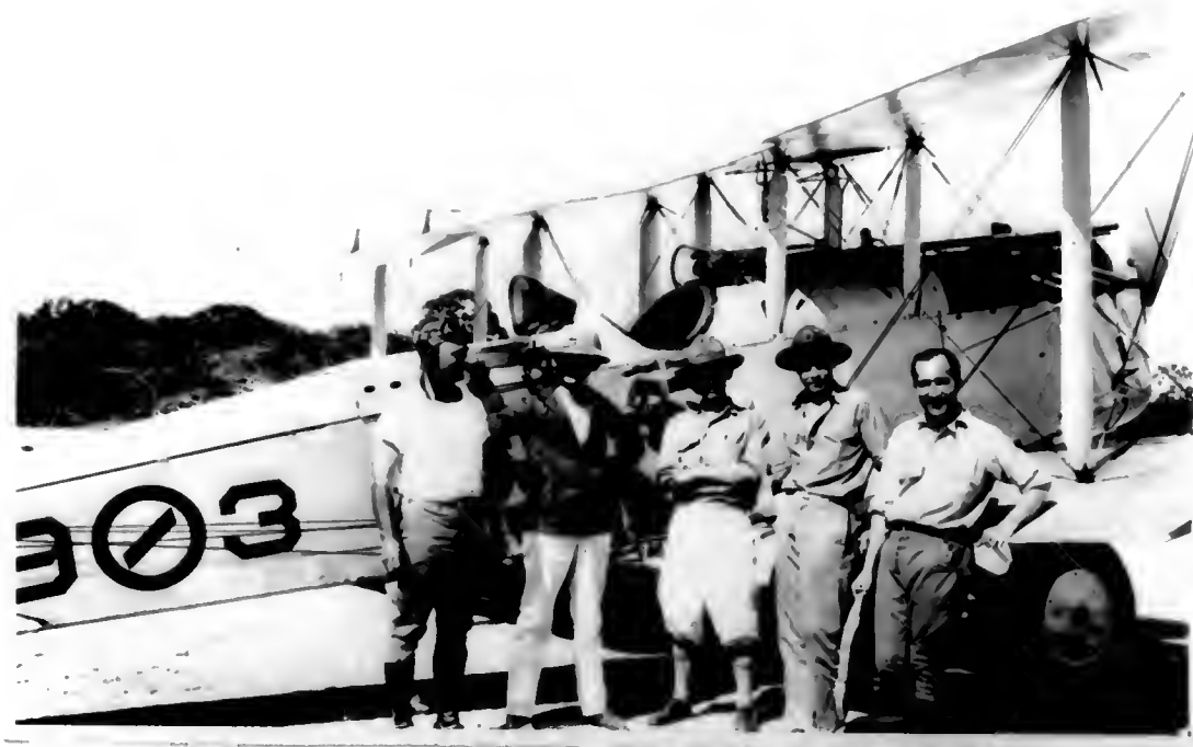
Aerial survey over Haiti. Tom Gill to the right.
