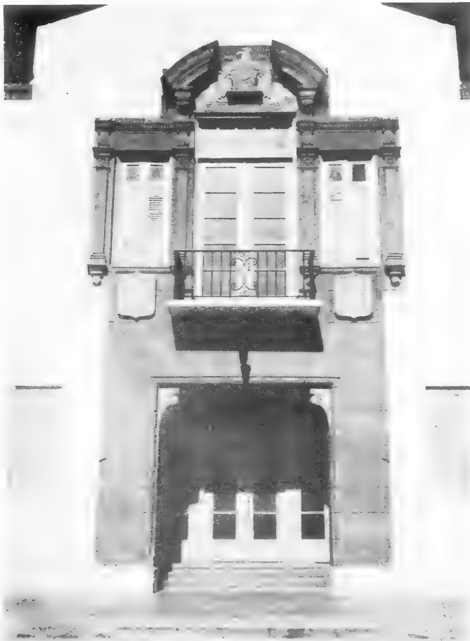
Top: Tropical Forest Experiment Station's new office and laboratory building. Bottom: A close-up of the entrance feature.
