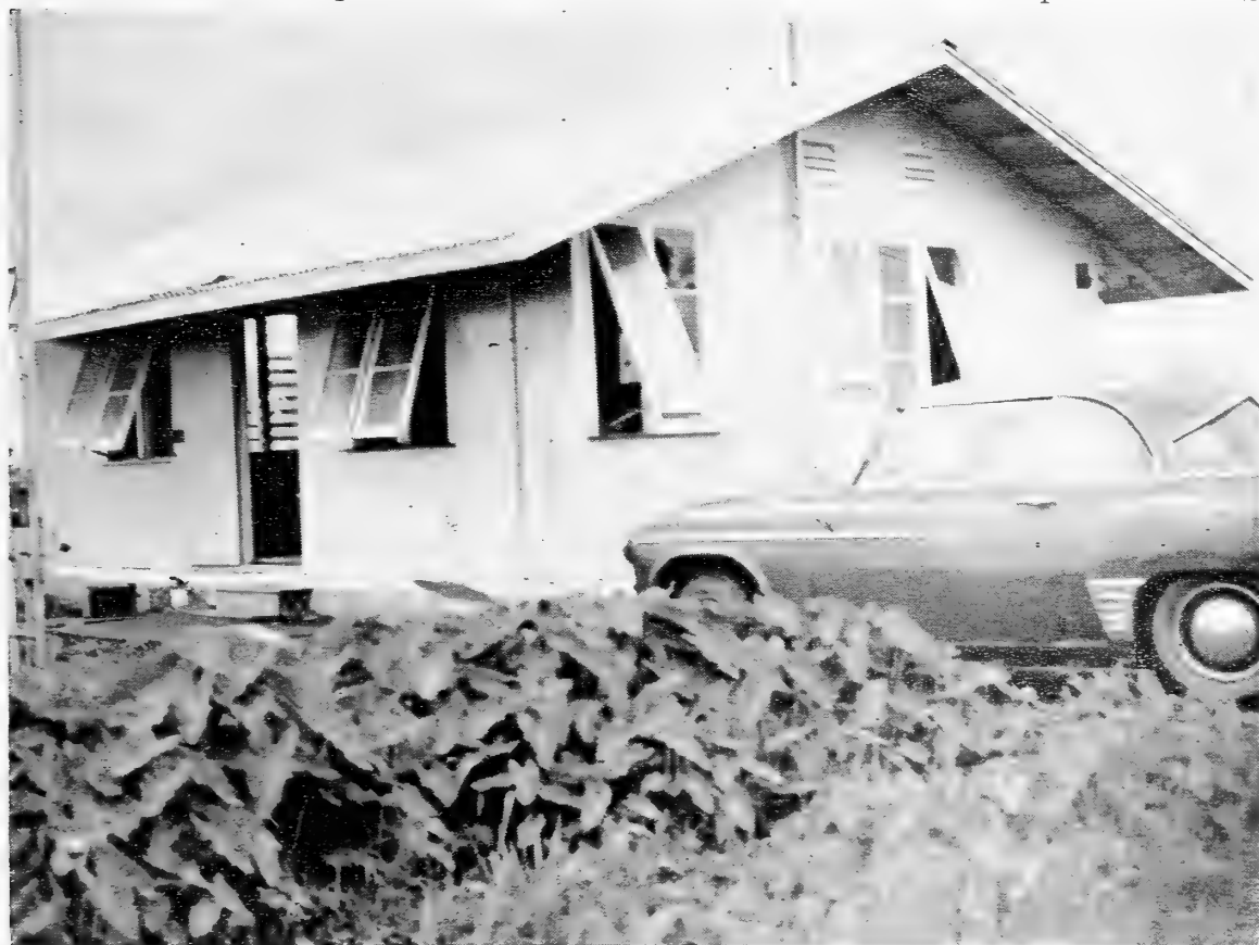
Figure 4. — Prefabricated house, British Guiana Timber Corporation.
