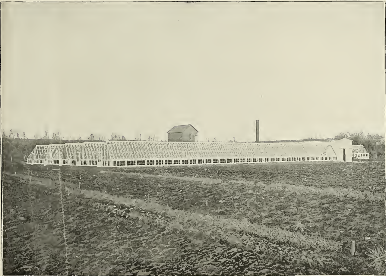
GREENHOUSES. GENERAL VIEW FROM SOUTH WEST CORNER.
