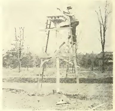
Fig. 712.—ADDING THE SECOND STORY.
