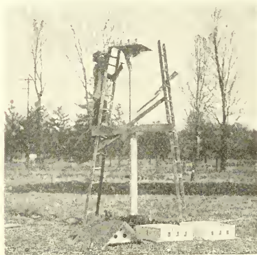
Fig. 711.—FIRST STORY IN PLACE.
