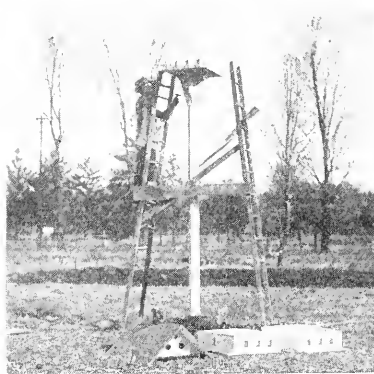
Fig. 711.—FIRST STORY IN PLACE.
