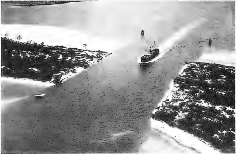
a. Inlet channel to Panama City Harbor prior to jetty construction
