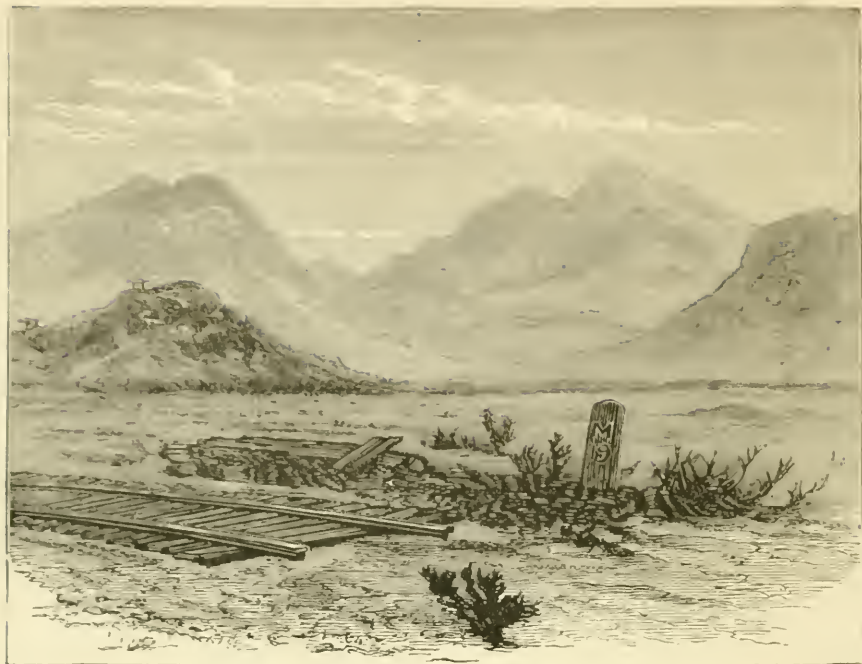
END OF THE SUAKIM RAILWAY AT OTAO.
