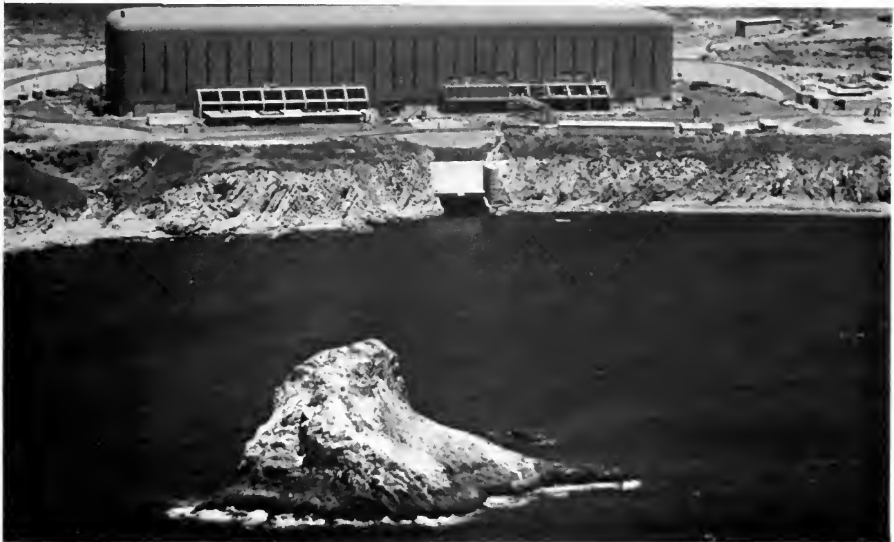
Diablo Rock off of Diablo Canyon Nuclear Power Plant
