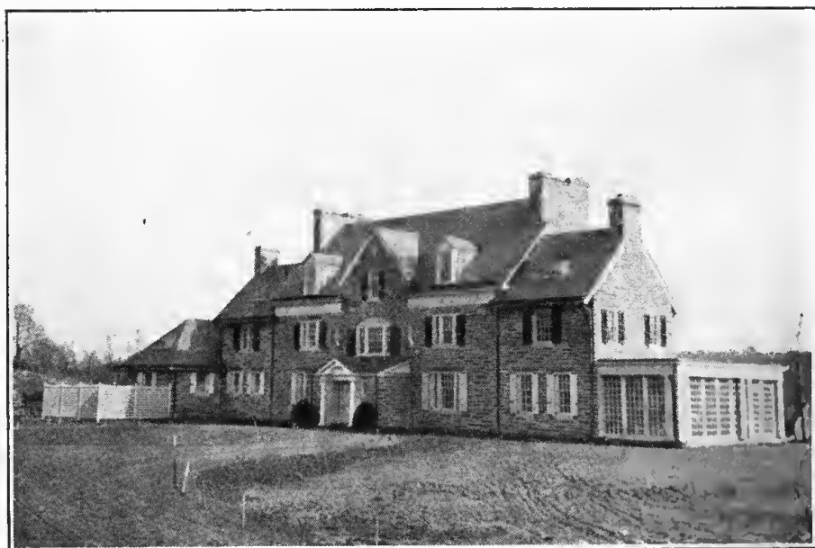
The House as the Builders Left It in the Early Spring
