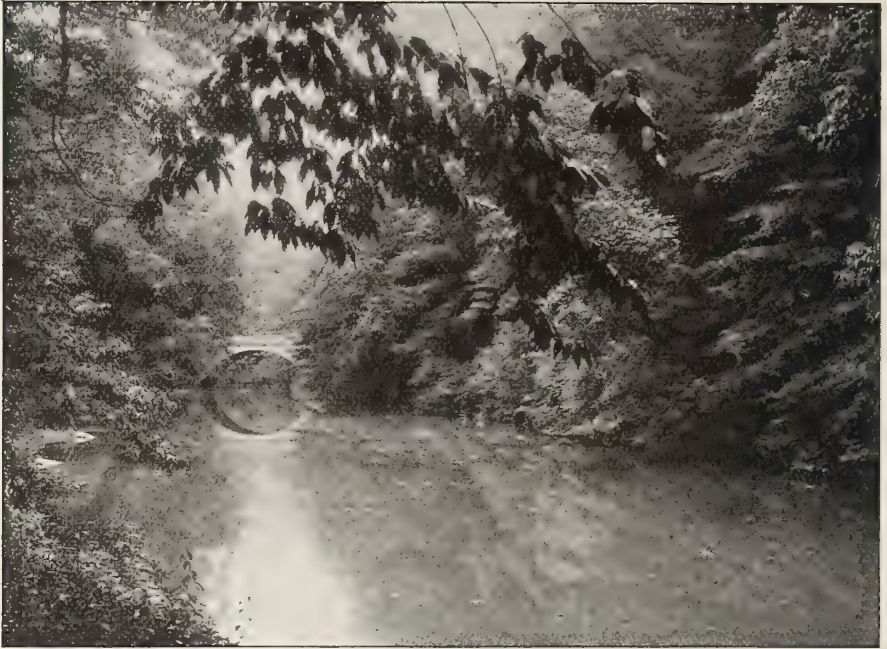
BRIDGE LEADING TO WISSAHICKON INN.
