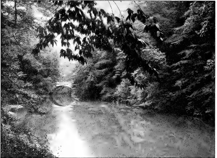
BRIDGE LEADING TO WISSAHICKON INN.
