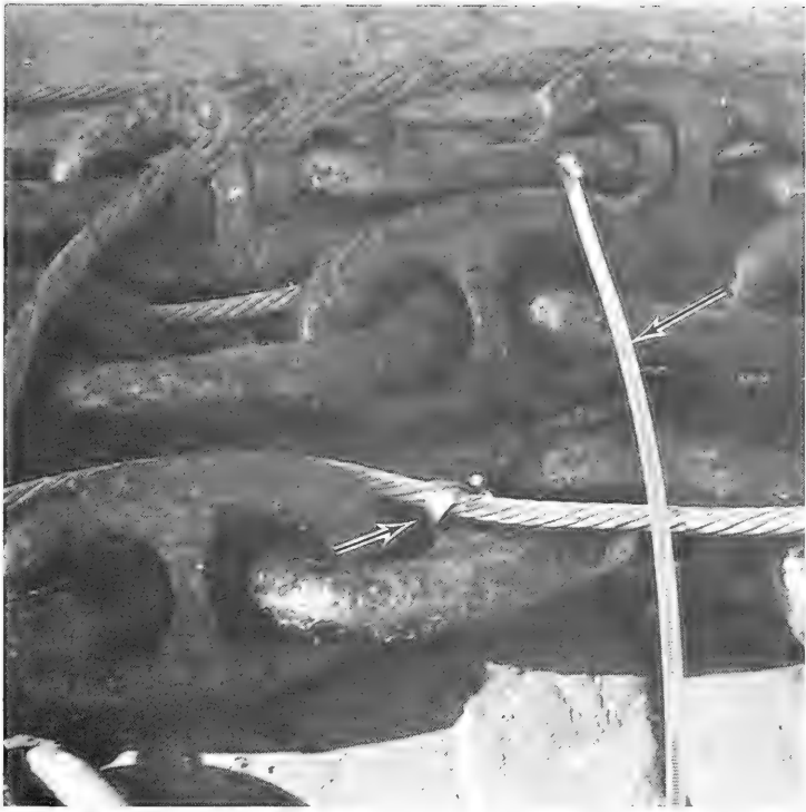
Figure 15. Cable clamped to chain link and a clamp shown prior to use.
