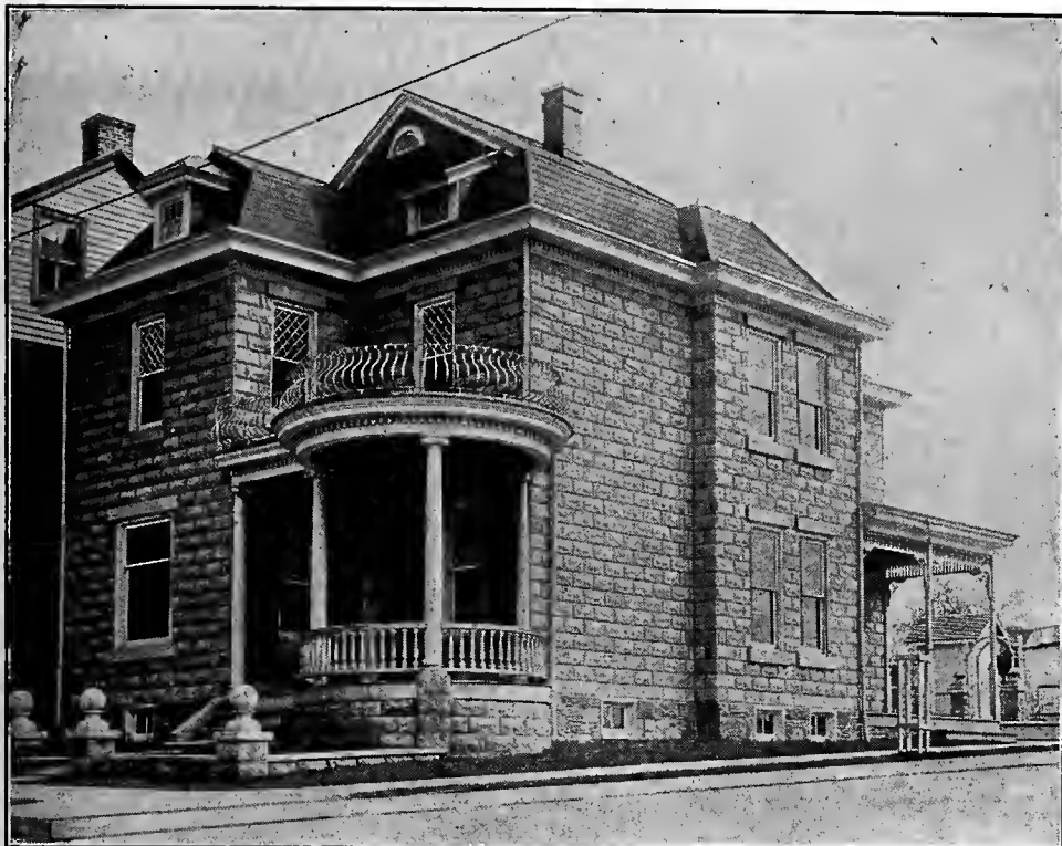
Residence of Michael Hein
