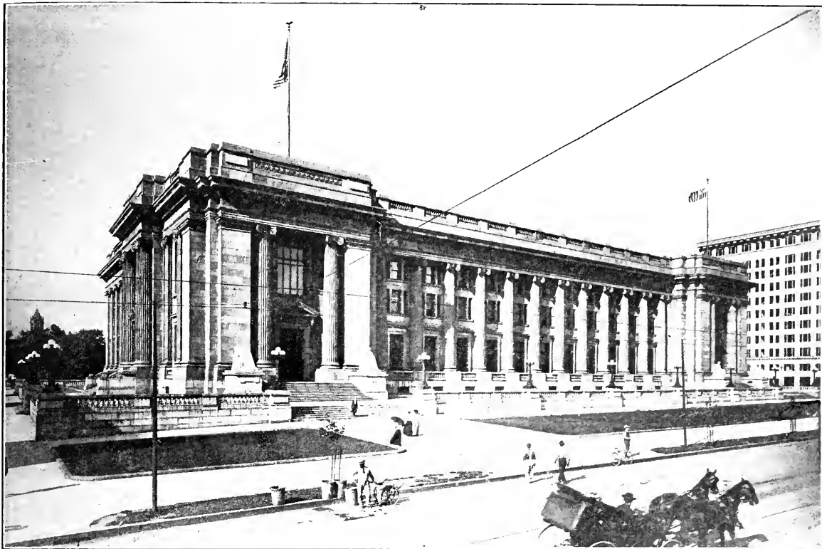
United States Court-House and Post-Office, Indianapolis.
