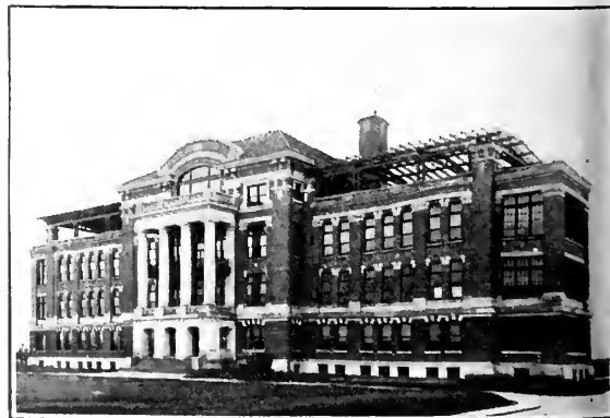
Robert W. Long Hospital, Indianapolis.
