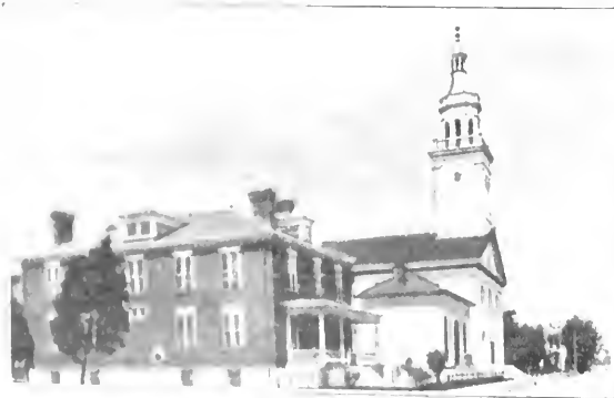
St. Francis Xavier Cathedral, Parsonage and Library, Vincennes.
