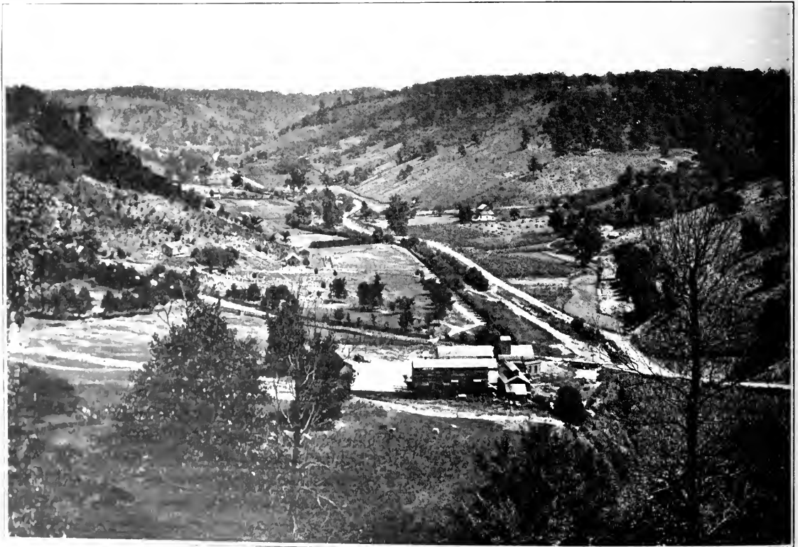
View of Canaan Road, Jefferson County.
