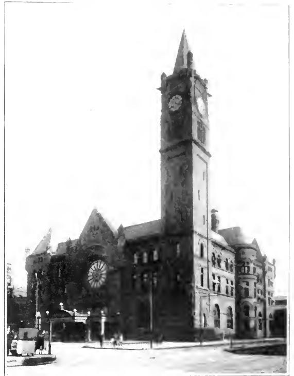
Union Station, Indianapolis.
