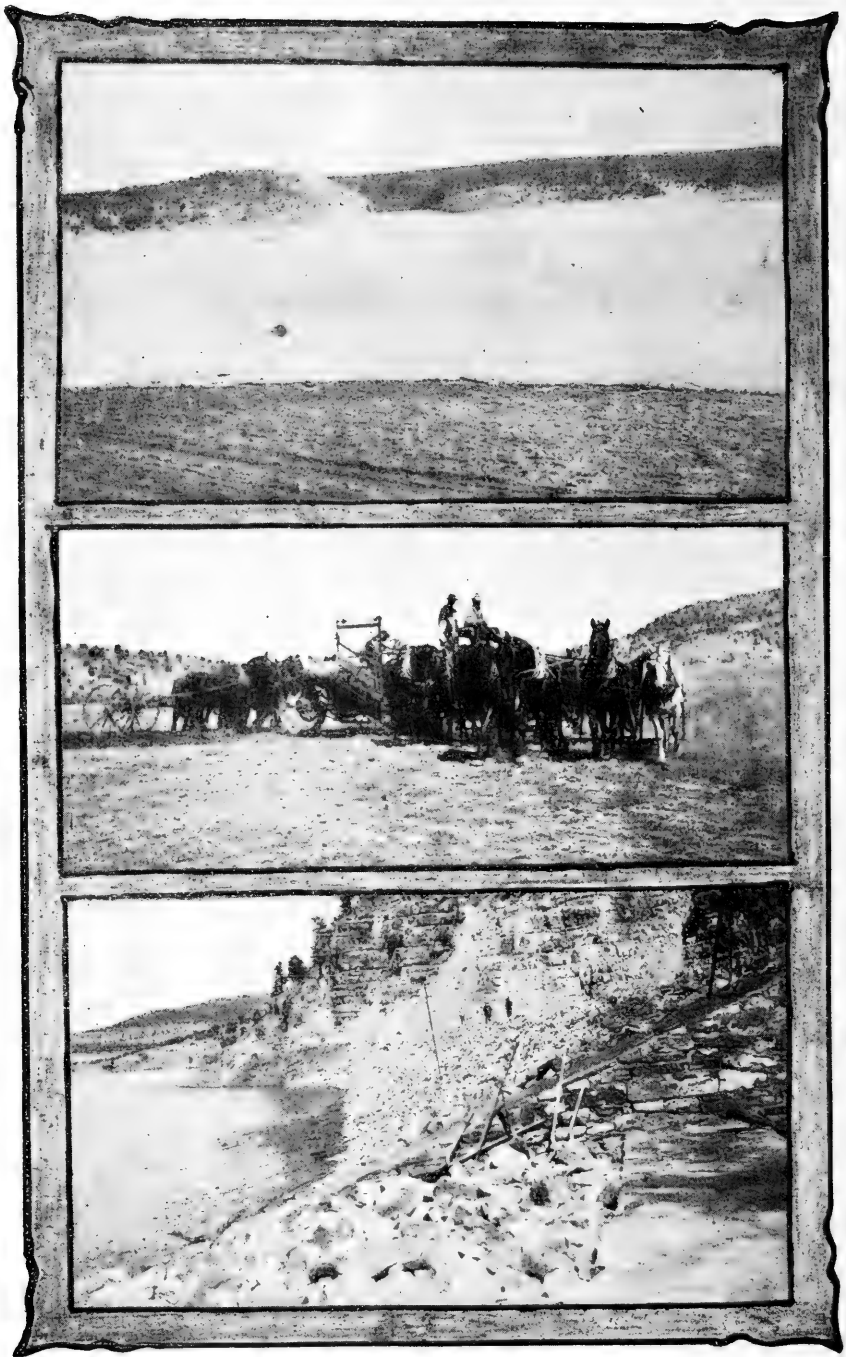
The Bluewater Project, Western Valencia County
