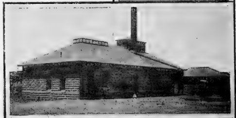
Water Works Plant
