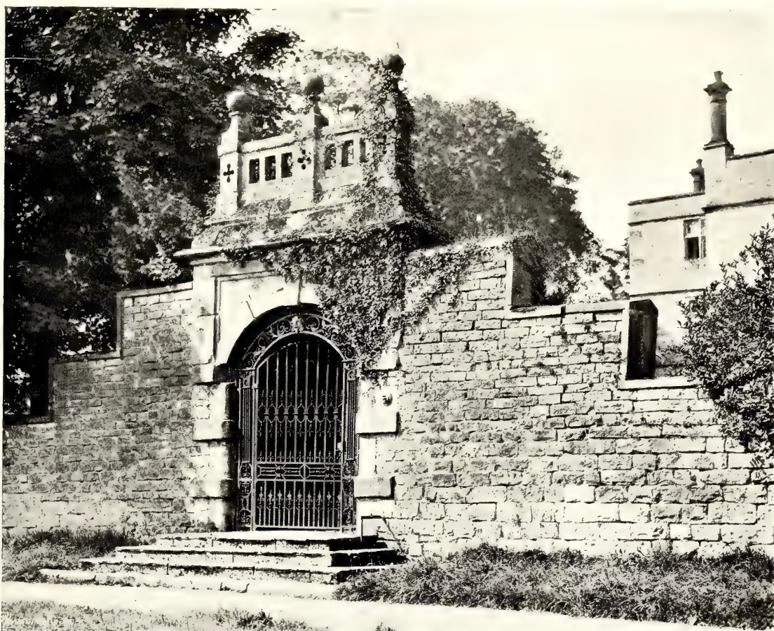
THE GATEWAY, TISSINGTON HALL, DERBYSHIRE.
