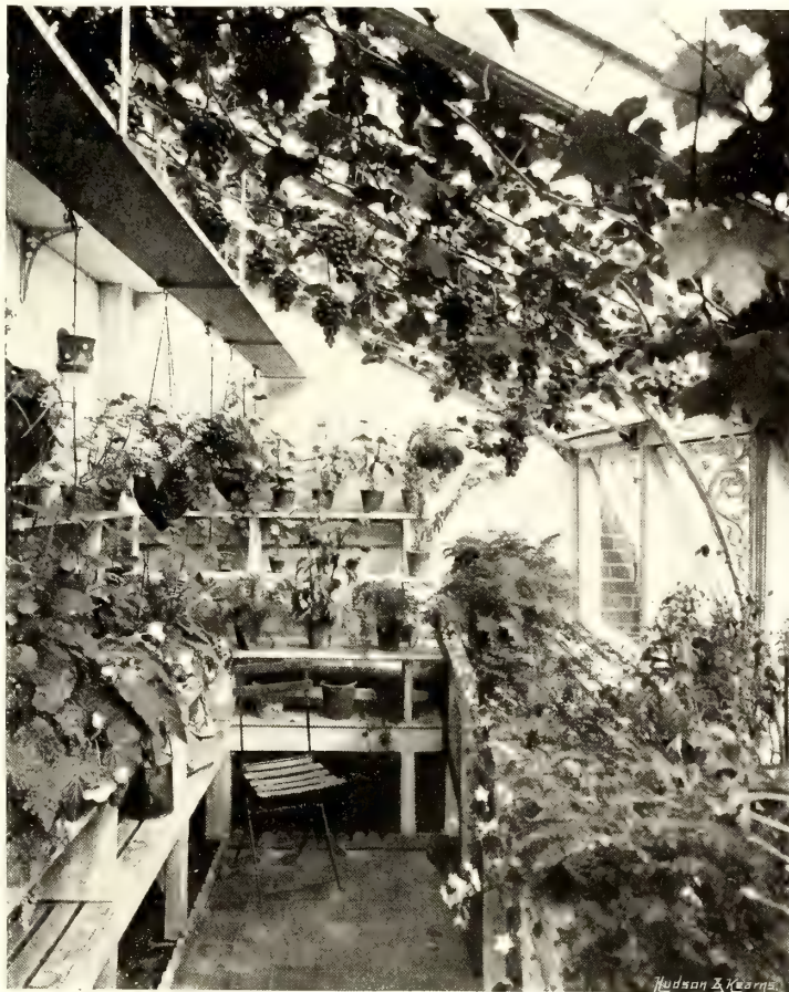
A VILLA VINERY AND GREENHOUSE.
