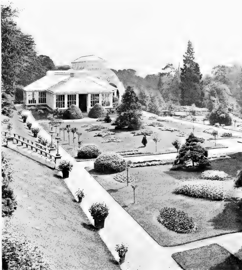
THE GREENHOUSES AT STREATHAM HALL, EXETER
