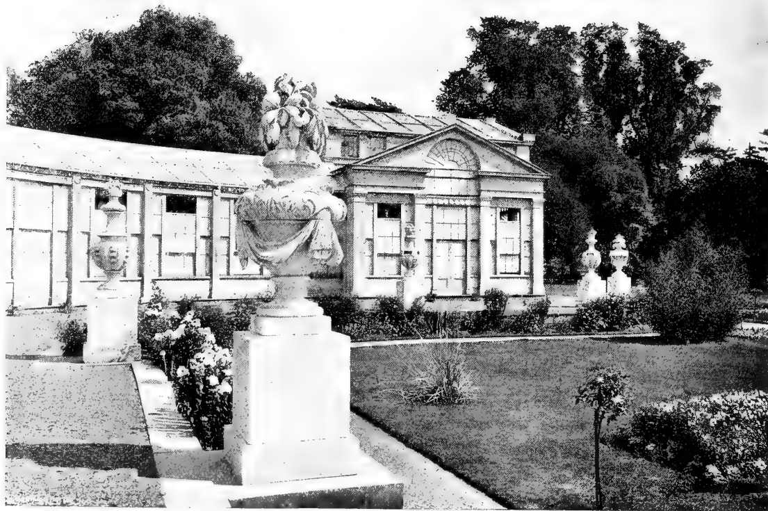
CONSERVATORY AT SYON HOUSE, MIDDLESEX.
