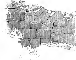
Cyclopean Masonry.—Walls of Assos, in the Troad. (From papers of the Archaeol. Inst. of America.)
