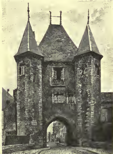
Gate-house.—Porte de Joigny, Vitry, France.
