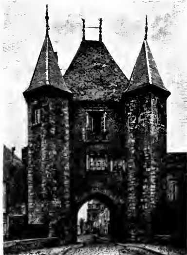
Gate-house.—Porte de Joigny, Vitry, France.
