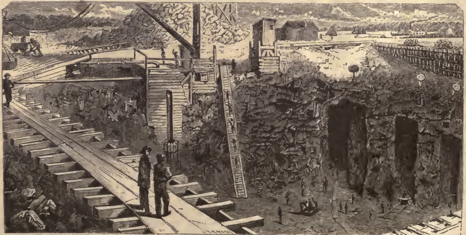
VIEW OF SHAFT FROM COFFER-DAM.
