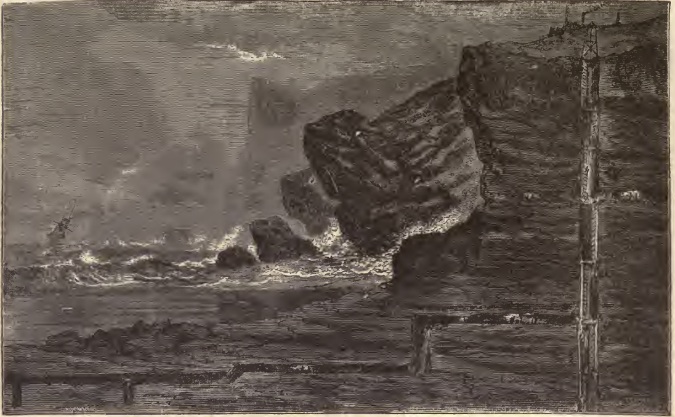
TIN MINE AT CAPE LAND'S-END, CORNWALL, ENGLAND—EXCAVATED UNDER THE SEA.
