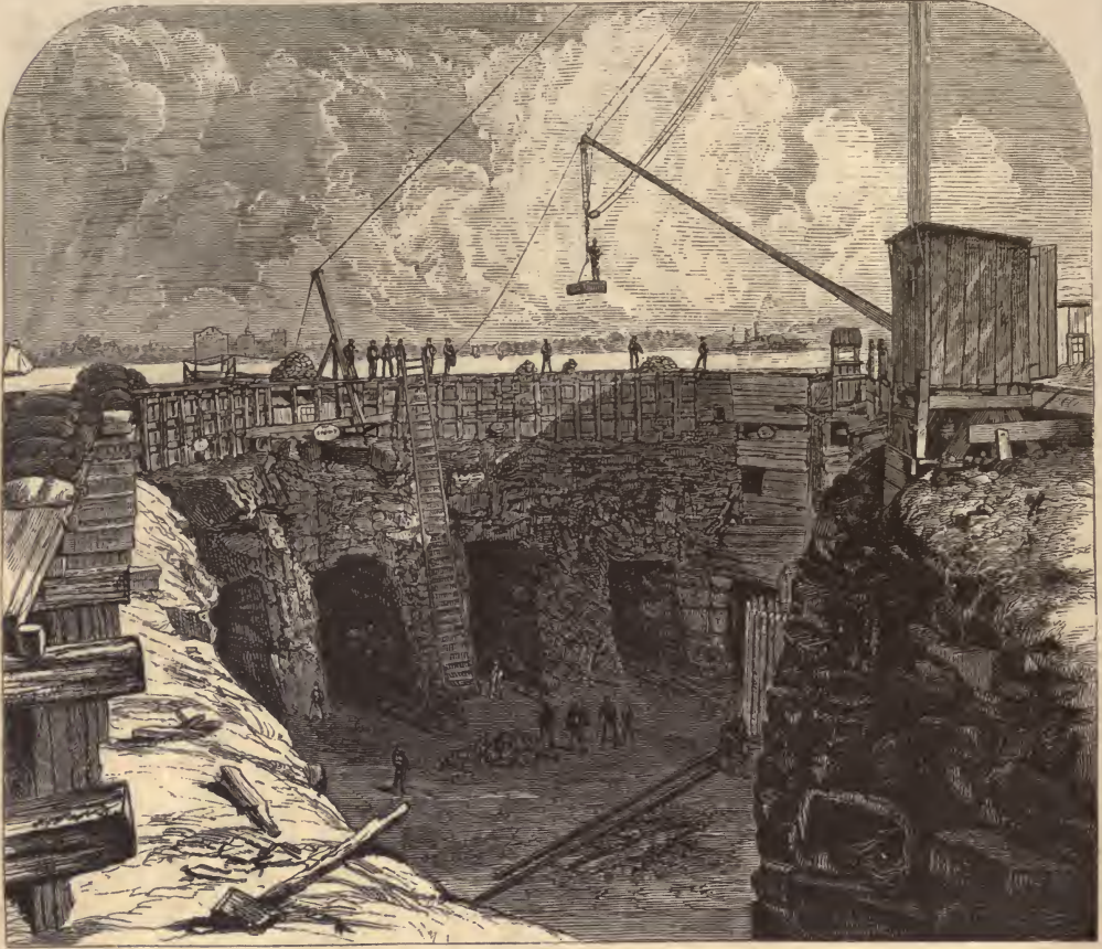
THE SHAFT, LOOKING EAST.
