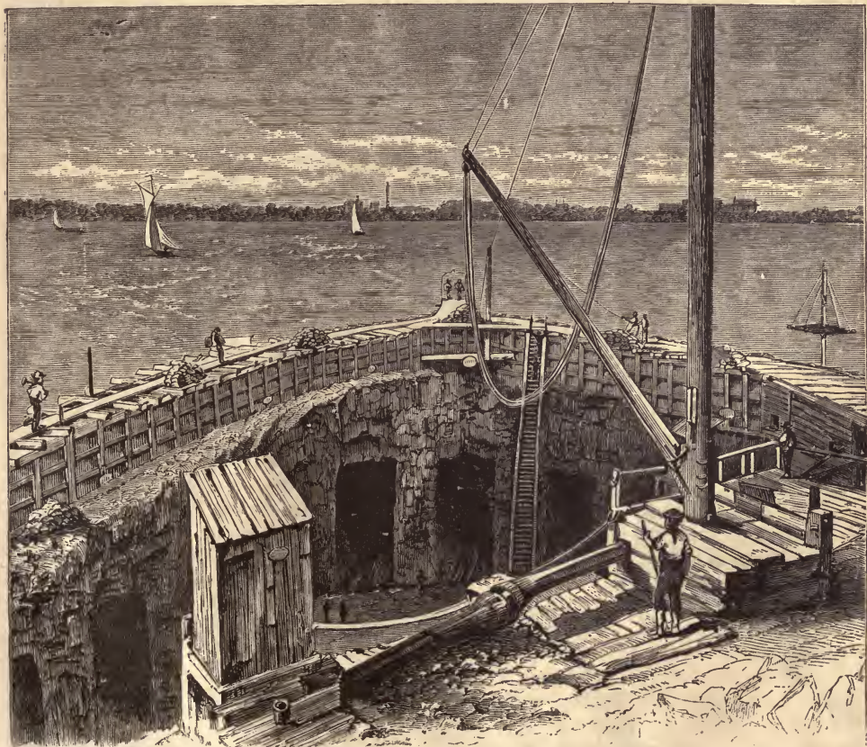
VIEW OF COFFER-DAM, LOOKING EAST.
