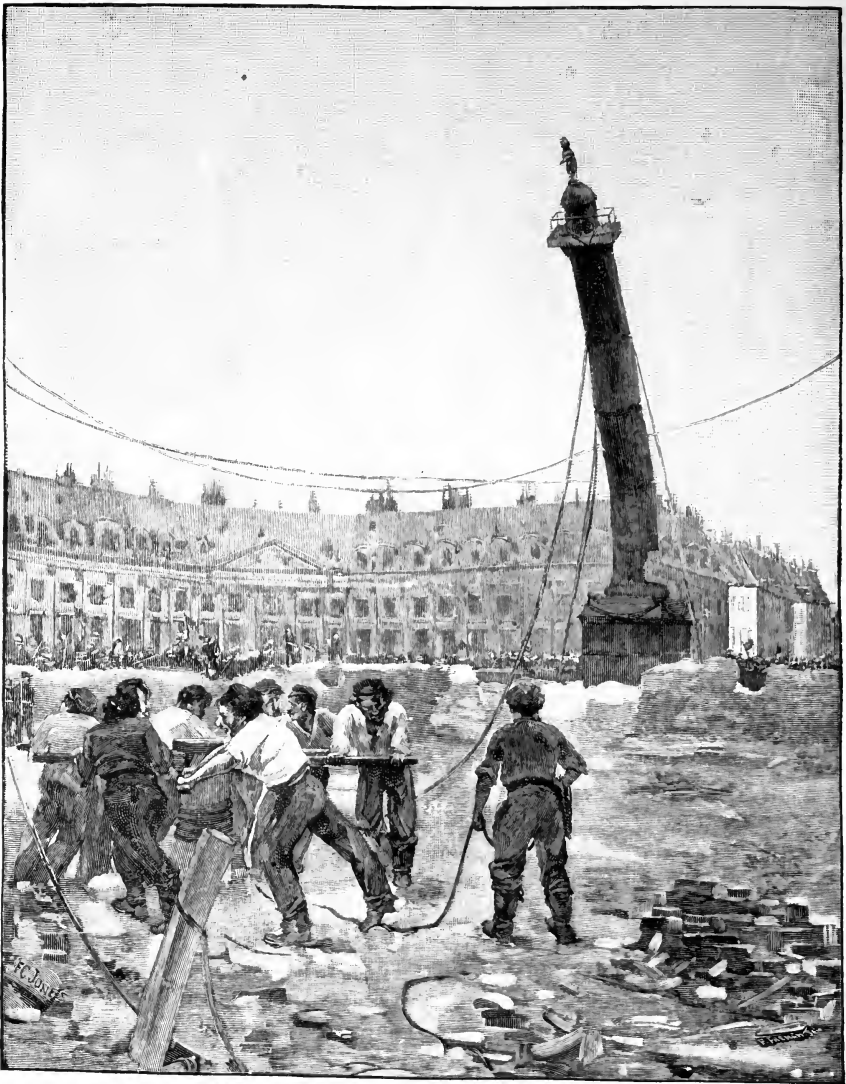
PULLING DOWN THE VENDÔME COLUMN.
