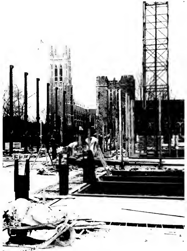
The construction of the new Administration Building, which completes the quadrangle, is fascinating to students.
