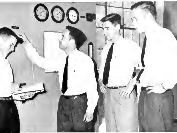
Try your hand at working this gem of a switchboard. Now you too will be a Pi Tau Sig.
