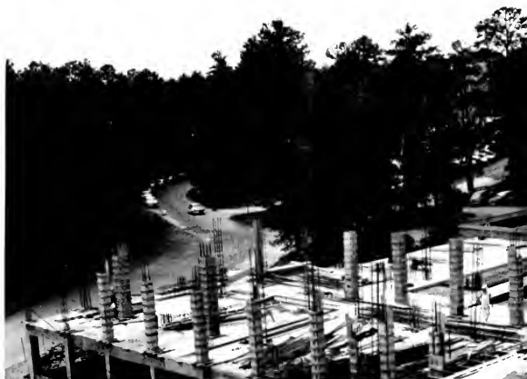
One of many construction projects on Duke campus is the new, three and one-quarter million dollar additional wing being added to the hospital.
