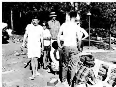
PiKA construction company.
