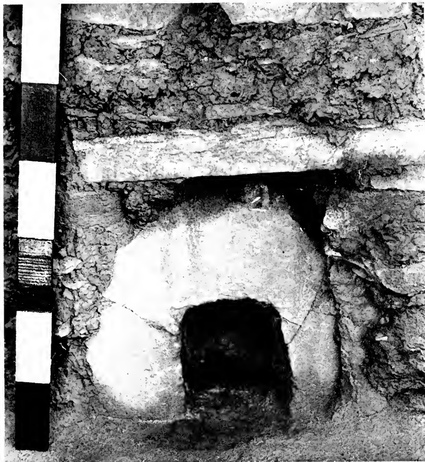
FIG. 9. Ventilator opening framed with horseshoe-shaped slab in east wall of Room 11. Meter stick at left.
