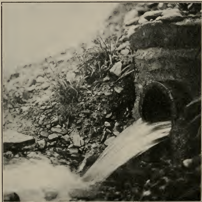
FIG. 38.—Waste water. Outlet of drain tile. (Elliott.)
