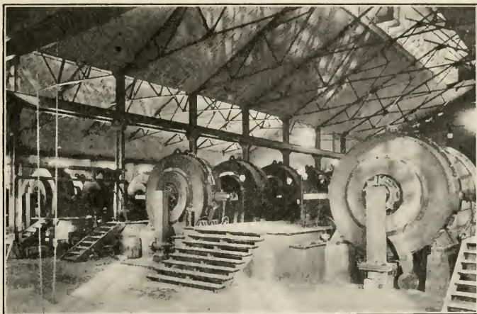
FIG. 47.—Manufacture of calcium nitrate. Interior view of furnace house at Notodden, Norway.
