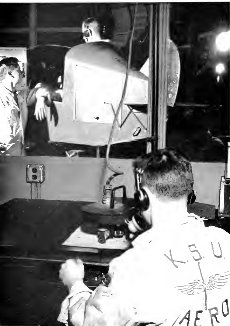
FLIGHT INSTRUMENTS in the Link trainer are controlled from a glass-paneled booth in aeronautics.
