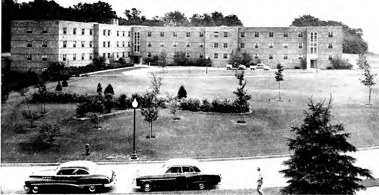
STOPHER HALL, perched on a rise above the Commons, is built in an "L" shape, and accomodates 275 men.
