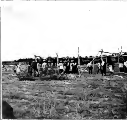
FIG. 44. Erecting the lodge.
