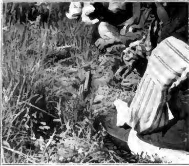
FIG. 10. The pipe-tampers and new earth.
