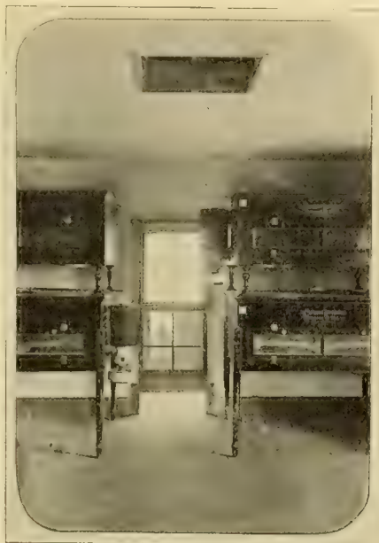
Ventilating Openings in Ceiling and Window in Incubator Room on Jordan Poultry Plant.
