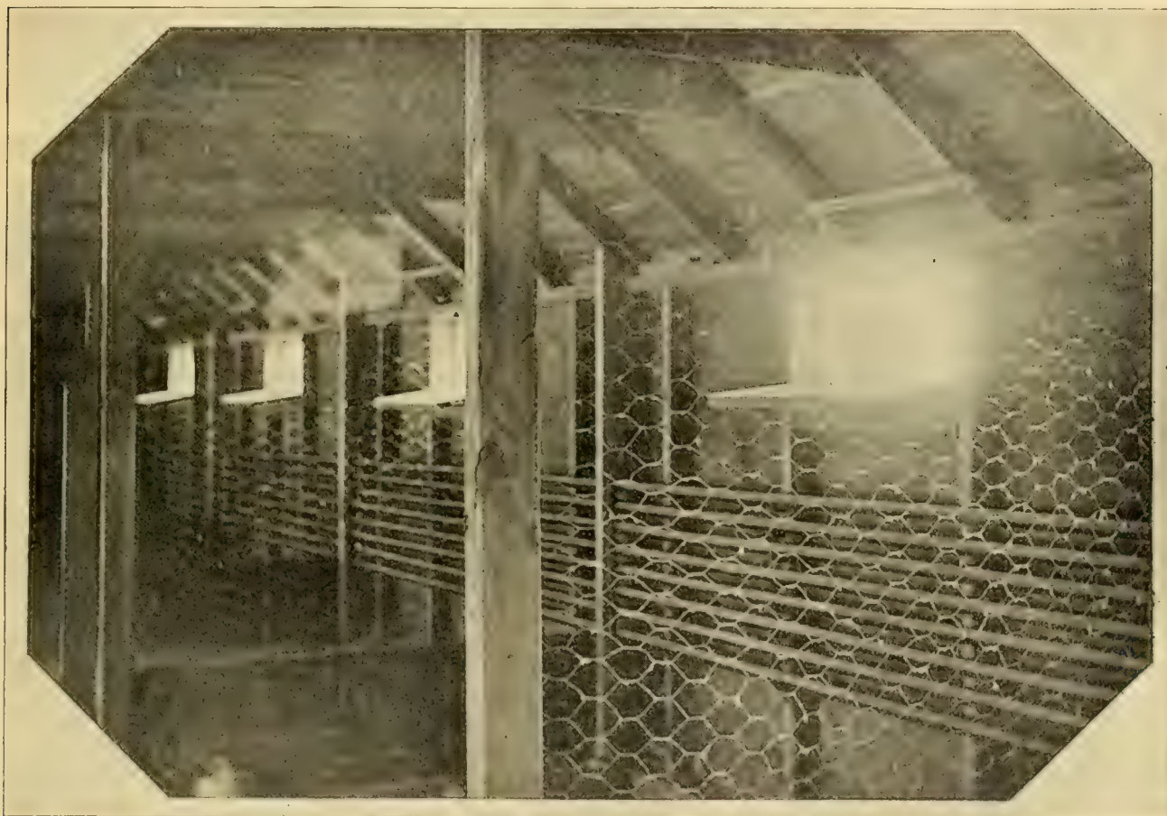
Interior of a Brooding House on the Jordan Poultry Plant, Showing Pipes for Warming the House.
