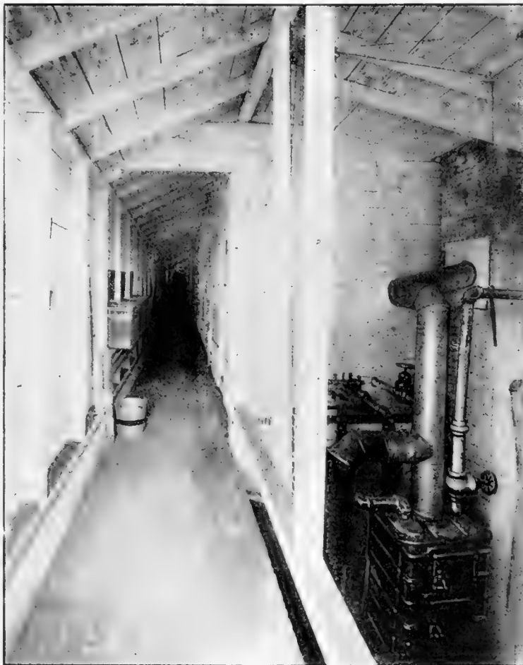
The Heater which Feeds the Pipe Systems In a New Jersey Brooding House.
