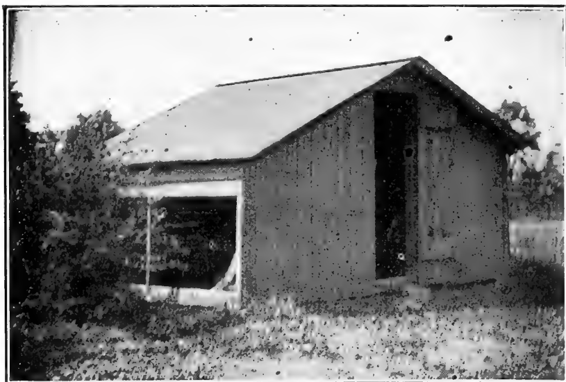
Figure 5—Open Front House, Without Curtain or Glass
