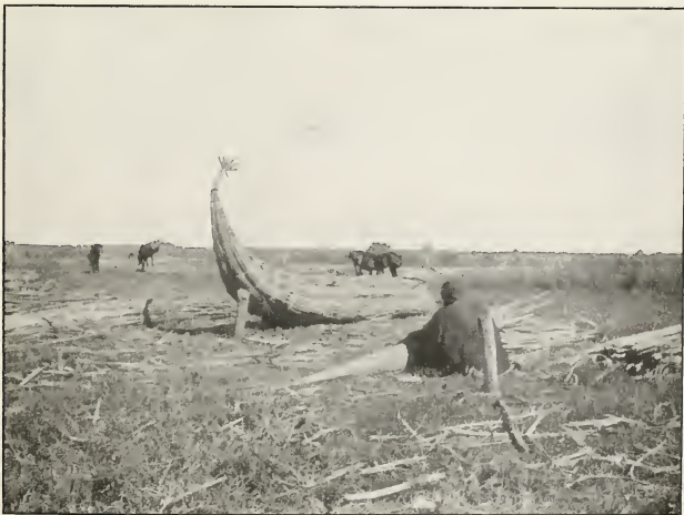
A Buduma Canoe in the Process of Construction.
