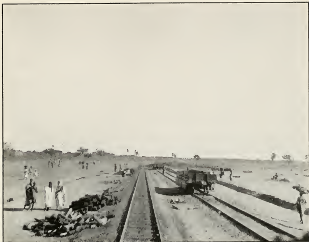
New Railway Line at Kano.
