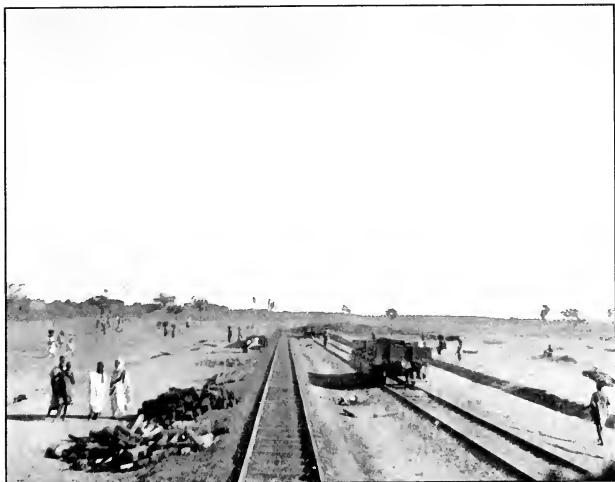
New Railway Line at Kano.
