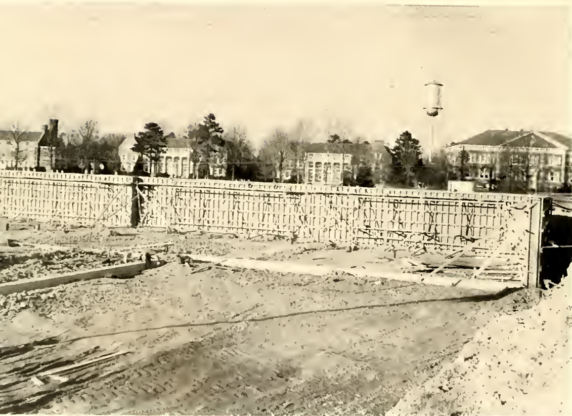
... science building under construction ...
