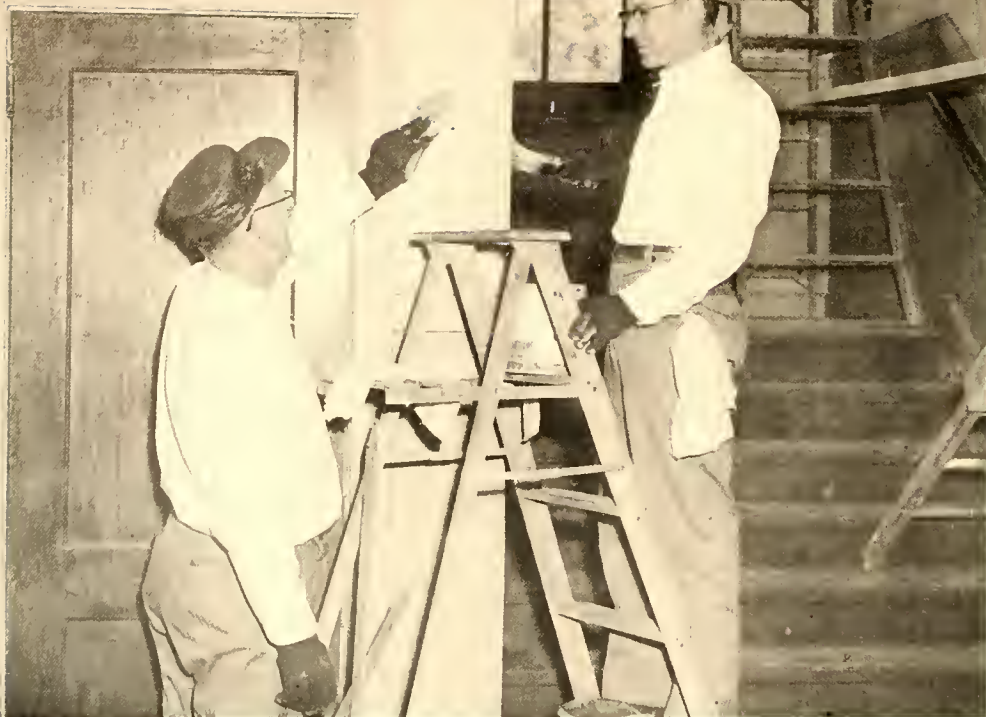
Boiler break-down . . . "Where's the plumber's friend?" . . . A jeep refuses to move . . . constant paint jobs.
