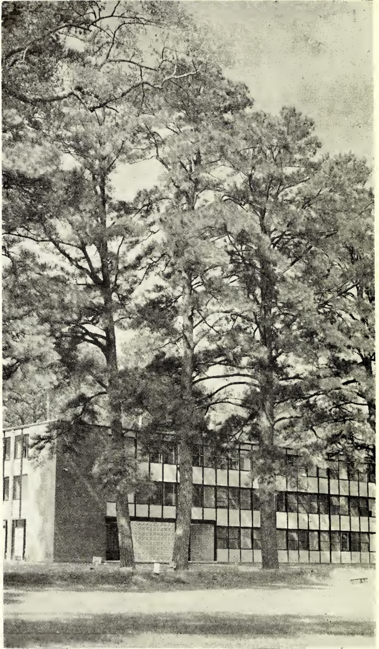
One of the latest additions to the Chowan College campus is a new dormitory for men. Modern and functional in every respect, it provides highly desirable living quarters for 116 male students.
